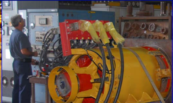
Testing 1500-kW Generator at Full Load
