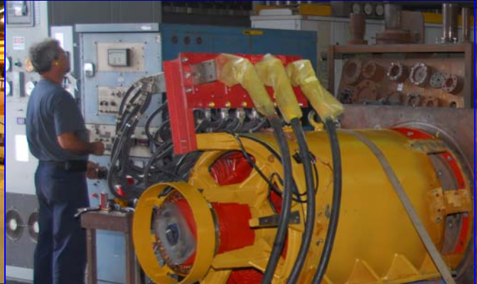
Testing 1500-kW Generator at Full Load
